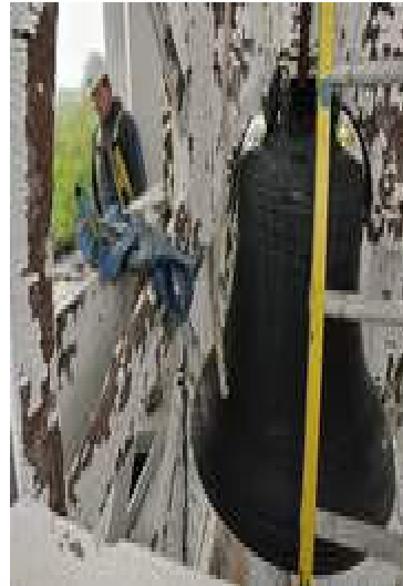
Supervisor Matthew Buckley of Murray Brothers Construction of Leominster works around the 1060-pound Paul Revere bell in the steeple of the Bulfinch church on the Town Green. (T&G Staff/RICK CINCLAIR)
