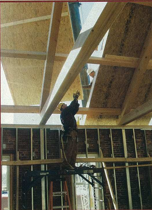
Workers guide an 8-foot by 24-foot roof panel into position on purlins.
