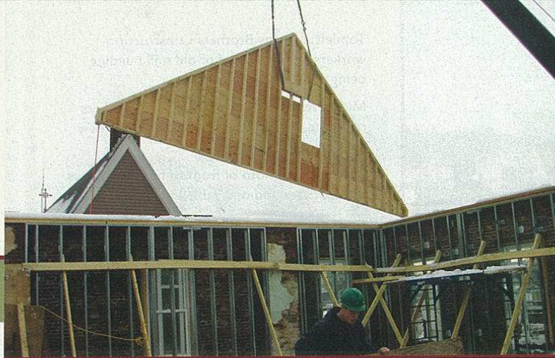
For lack of space, gable end walls were fabricated on third floor, then lowered to alleyway at street level until ready for final positioning.
